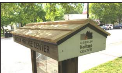
Even the tiniest roofs need some TLC. Thanks to board member Nikki Smith-Hignite for putting new cedar shakes on the Main Street kiosk.
