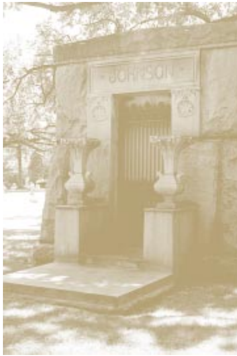
Large slabs of granite make up the ornate Johnson Mauseleum. The door and grillwork are bronze.
