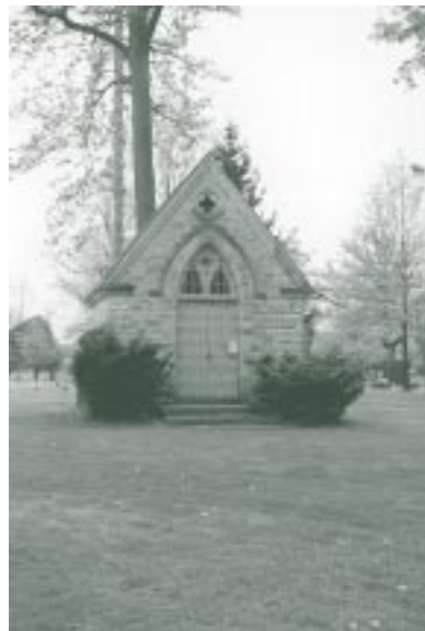
Receiving vault built in 1887. It is now used for storage.
