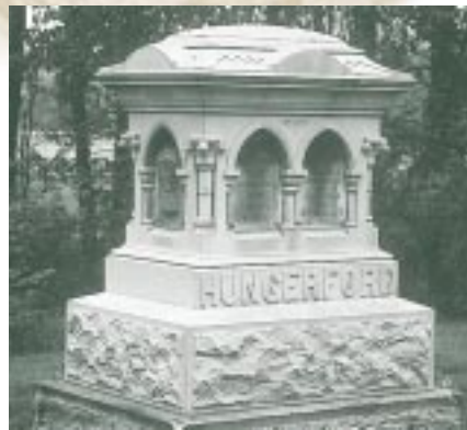
Sec. D. The Hungerford monument is hollow, cast aluminum with a sandstone base. This style was popular in other local cemeteries but is the only one of its kind in Westwood.
